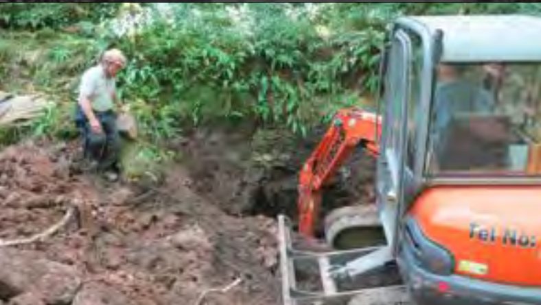
The digger in action - July 2013
