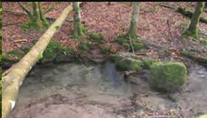
Longwood Main Sink, silted up and flooding - April 2013
