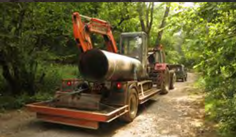
Digger and piping being transported to site - July 2013
