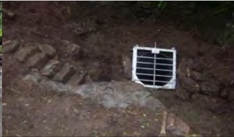
After: Longwood Valley Sink debris grill and gate
