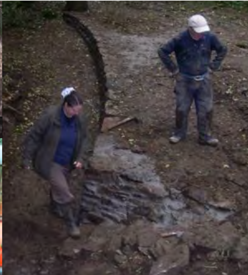
The permanent dam - September 2013
