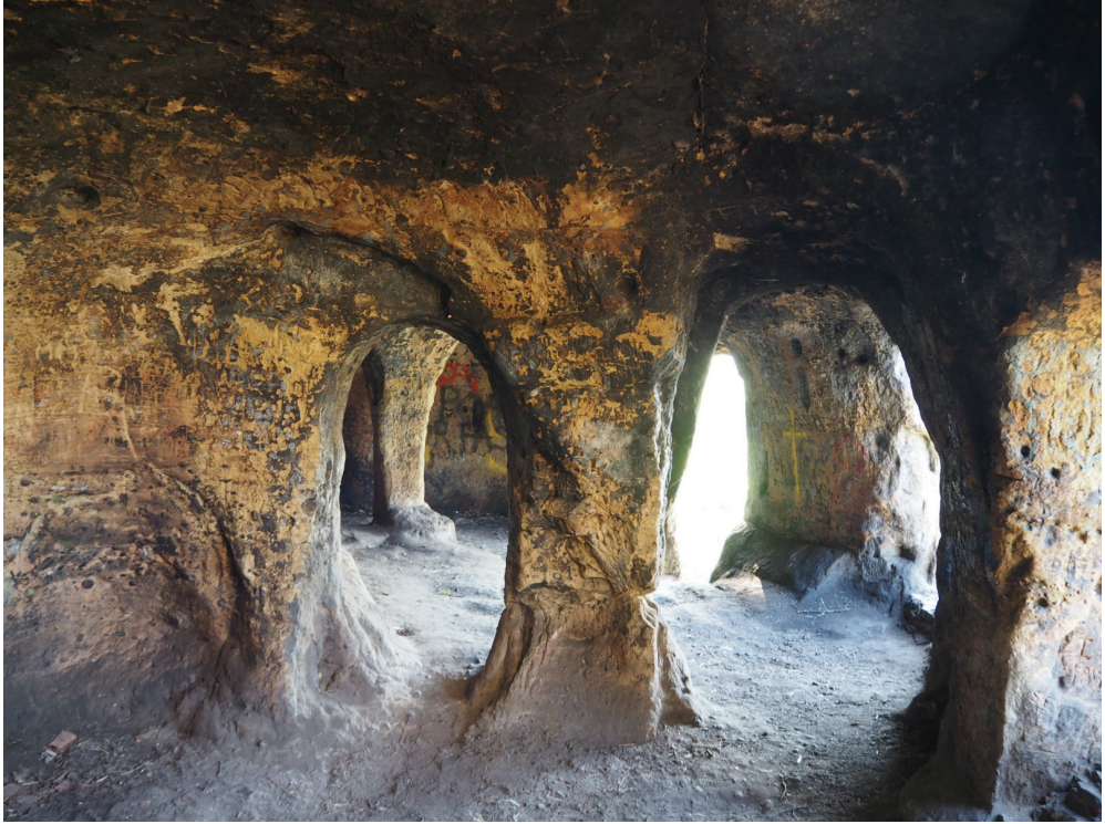
Figure 7. The pillar between Room A2 and A3, viewed from A3. The door is on the left and the opening on the right is the result of a later demolition, being punched through the thin wall of a former blind arch. The arches spring from a crude, but very obvious pilaster cap on what is now a column.
