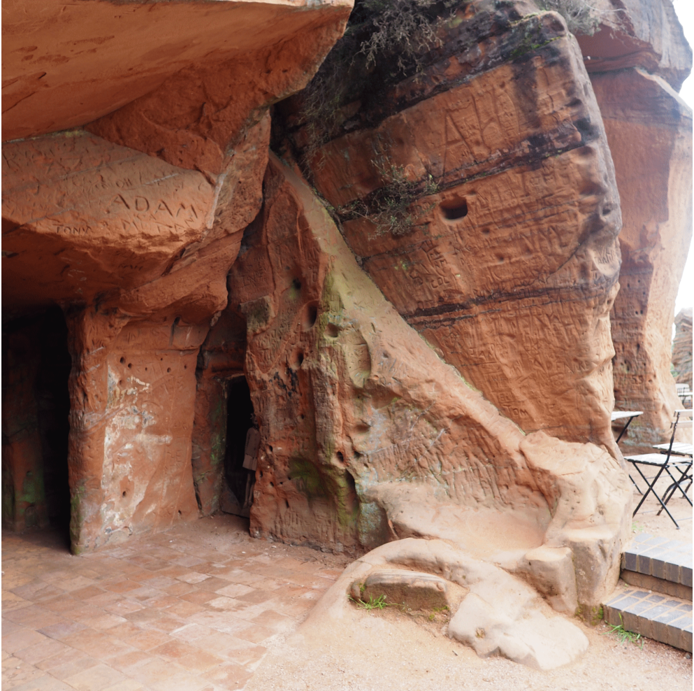
Figure 11. This fragmentary hearth in Room D 1 typifies the complexity of the site. A hearth with round back, sat next to a lost wall, with a (partly surviving) chimney above. A single joist pocket may indicate a smoke hood. At a later date the floor was lowered and a more simple hearth with brick chimney set to the front of the redundant hearth.
