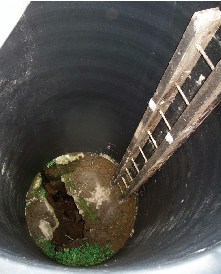
Figure 2. The newly installed entrance pipe at Polldonough South, B9a entrance.
